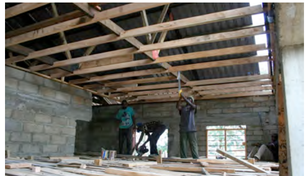
WORK BEING DONE ON THE CEILING OF THE RAFIKI KITCHEN
