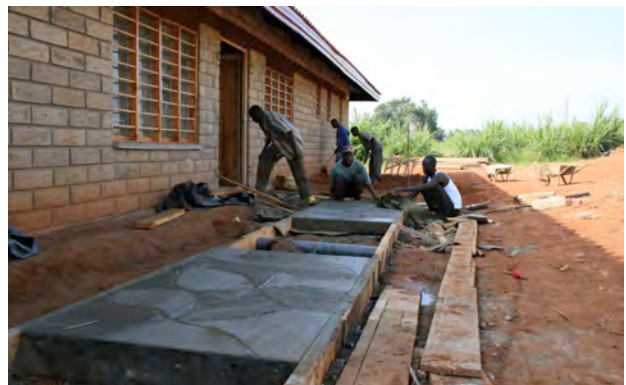
CEMENT BEING POURED FOR THE FIRST SIDEWALKS
