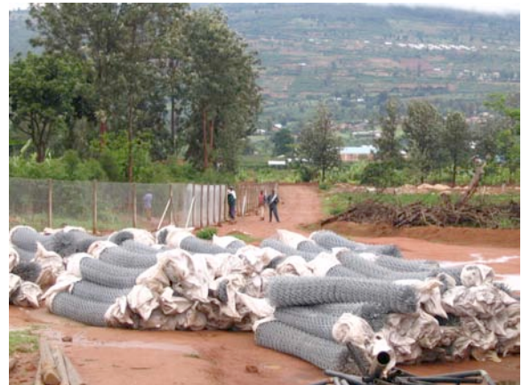
WIRE MESH FOR THE FENCH
