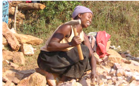
PERPETUE CHIPPING ROCK FOR FOUNDATION FOOTINGS
