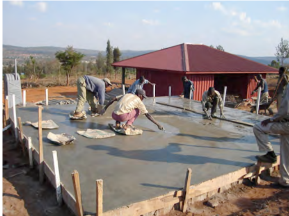
LAYING OF WATER-TANK SLAB
