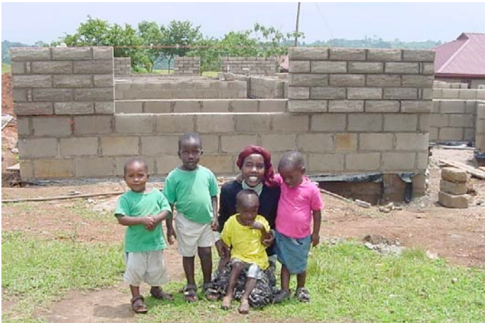
Mama Grace and her children in front of the school under construction
