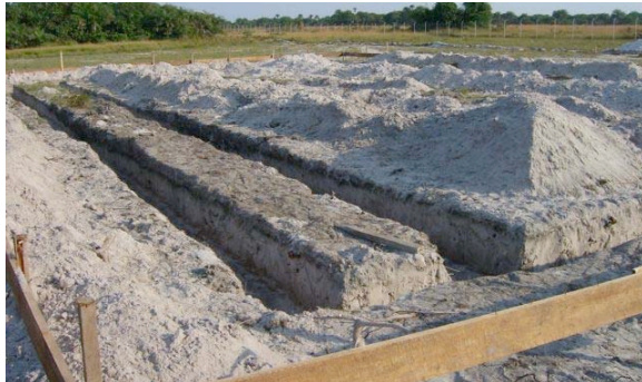
THE PRIMARY SCHOOL FOUNDATION, DECEMBER 2006.
