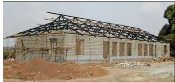
THE NEW DUPLEX UNDER CONSTRUCTION
