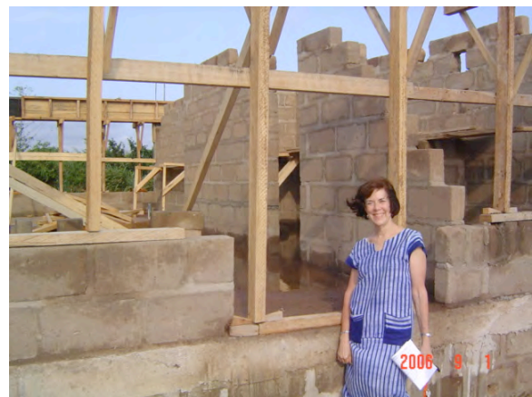
IN FRONT OF DINING HALL CONSTRUCTION
