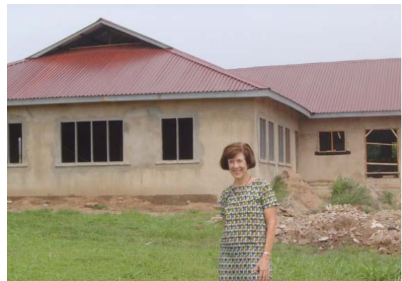
DINING HALL/KITCHEN/LAUNDRY BUILDING UNDER CONSTRUCTION
