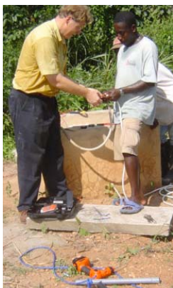
INSTALLING NEW WATER PUMP
