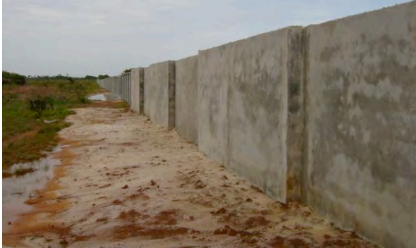
PROGRESS! RAFIKI VILLAGE WALL JUST BEFORE COMPLETION
