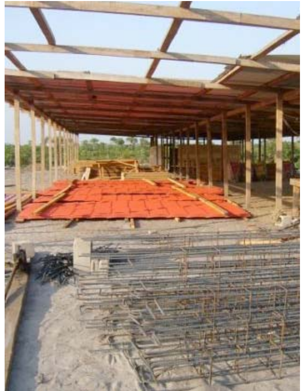
FOUNDATION STEEL AND ROOFING SHEETS
